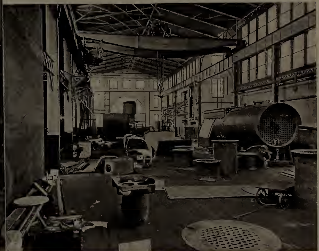
THE ATLANTIC WORKS, East Boston. Section of Boiler Shop, Interior.
